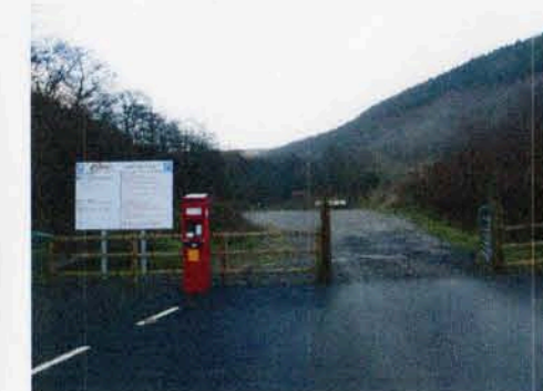
Visitor car park
