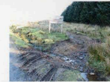
Off-road vehicle damage
