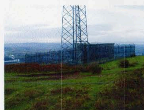
Telecom mast above Pontymoile
