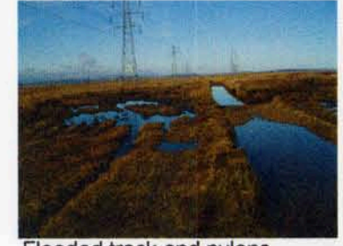
Flooded track and pylons
