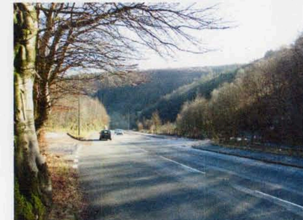
A472 looking east
